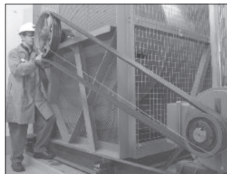
Using a string to check alignment
