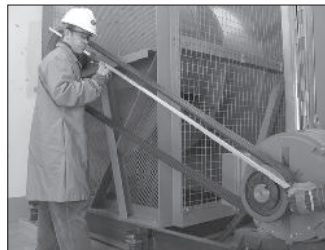
Using a straight edge to check alignment
