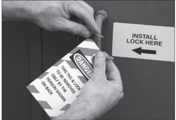
Turn off power, lock controls and tag
